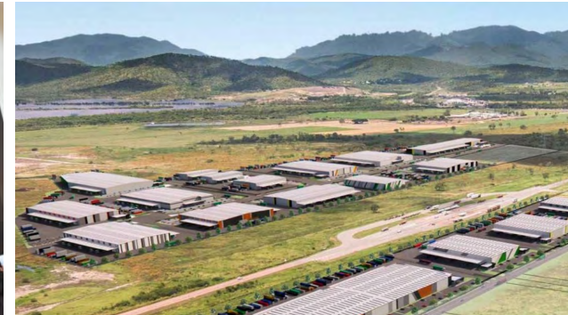
Queensland Resources Common User Facility Cost: $75m – processing plant for minerals
