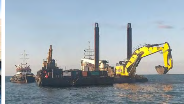
Townsville Port Expansion Cost: $232m – will cater to much larger ships
